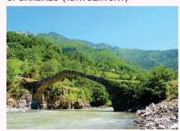
Dandalo Bridge is located in the village of Dandalo, near the Batumi-Akhaltsikhe highway. It is built on volcanic lime mortar rock. The piers are erected on a rock, on which scaffold holes have been preserved. The Dandalo arched bridge is one of the best examples of arched bridges in Georgia.
